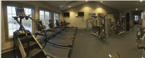
Pictured above is a photo submitted by David Gurulé of the gym reorganization in preparation for the final electrical work.
