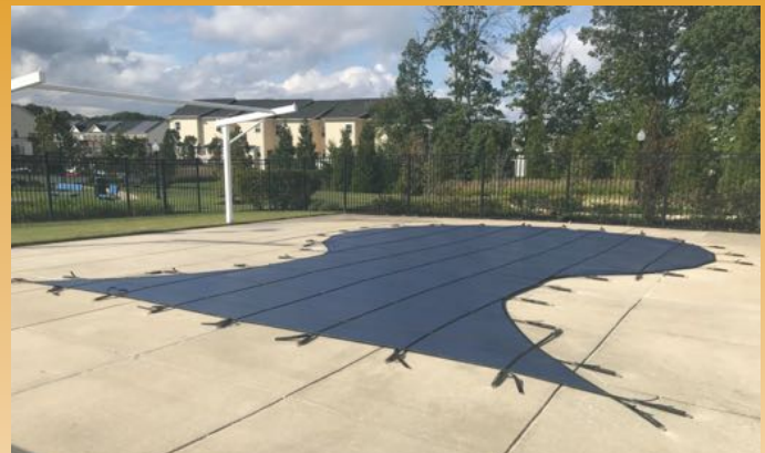
Pictured, freshly installed pool covers. Pool covers protect and prolong the pool's costly white coat from the elements and thereby extending the life of our pools' interior.
