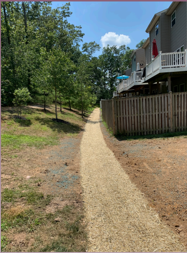
Pictured above, newly installed French drain on Coulbourn Corner to aid in drainage.
