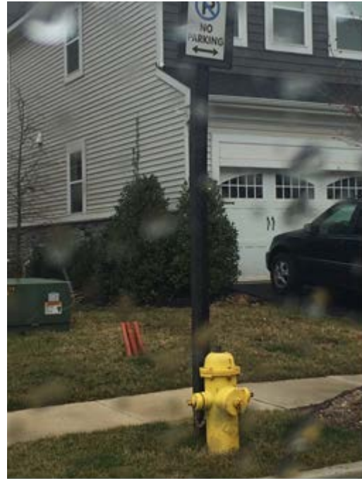
(Sign Post blocks hydrant wrench)
