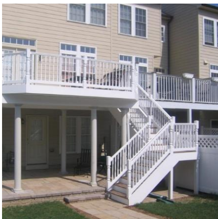
Staircase with landings example
