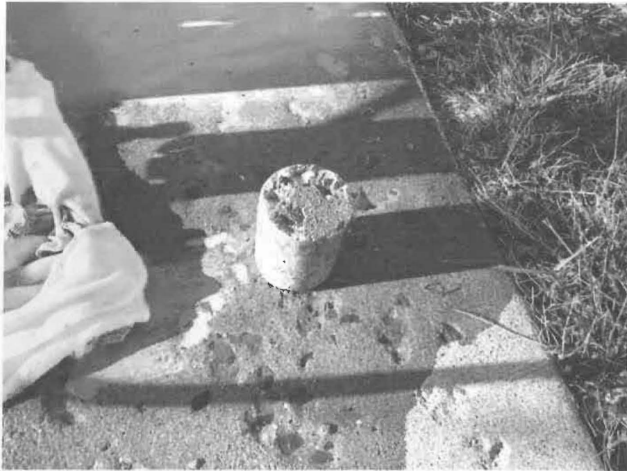
Photo 7 – Typical view of scaling in collected sample.
