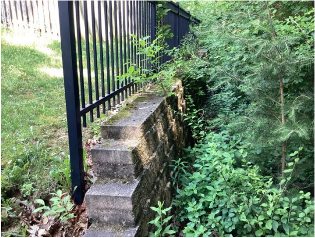
Retaining wall overview
