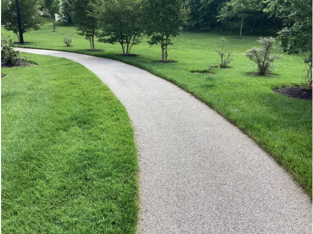
Asphalt pavement walking path overview
