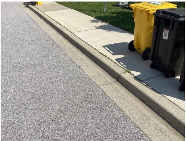
Concrete curb and gutter overview
