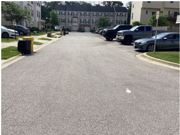
Section B and C pavement overview
