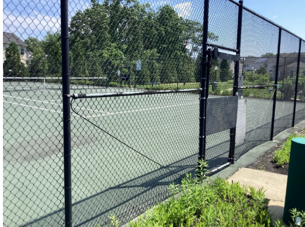
Tennis court fence overview
