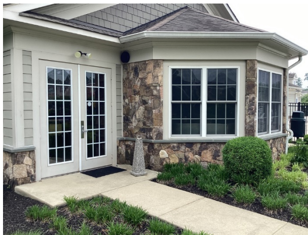
Clubhouse windows and doors
