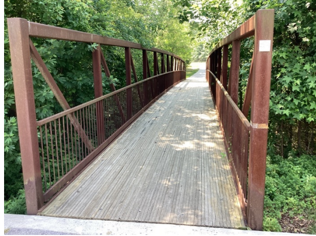
Pedestrian bridge overview
