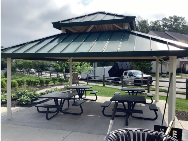
Archibald drive pavilion overview
