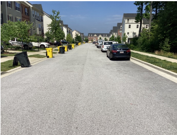
Section D and Oak Pointe pavement overview
