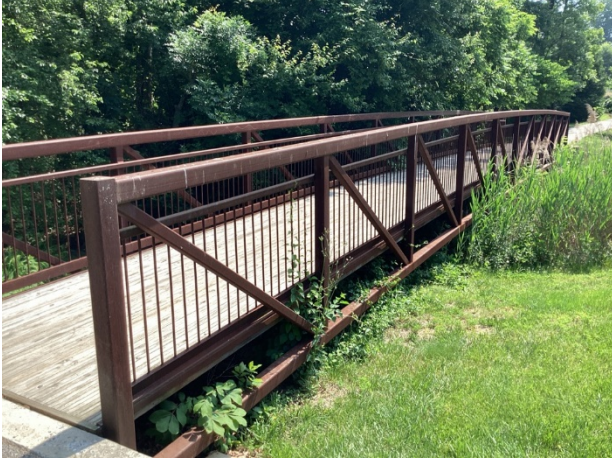
Pedestrian bridge overview
