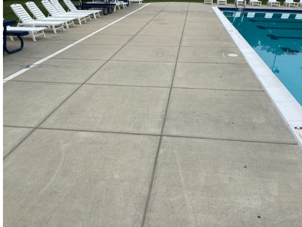
Concrete deck overview
