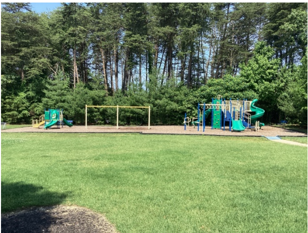
Mockingbird Circle playground overview Note: Finish deterioration.
