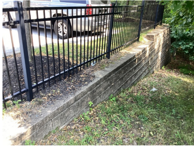
Retaining wall overview
