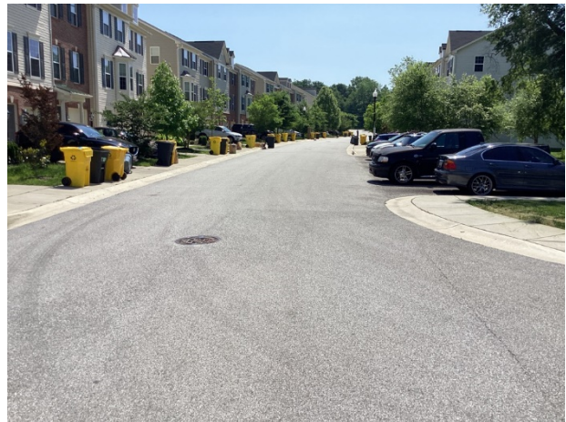
Section D and Oak Pointe pavement overview
