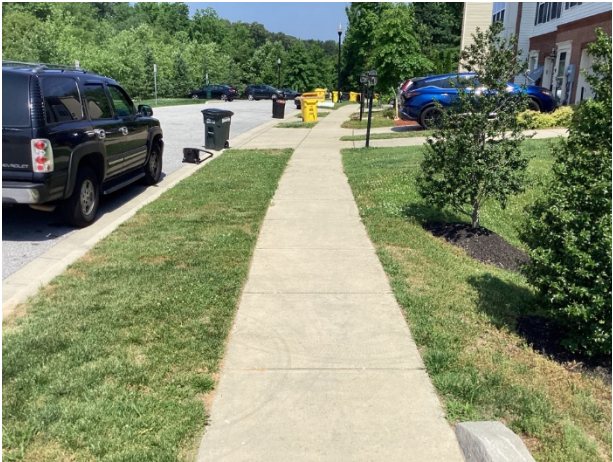
Concrete sidewalk overview
