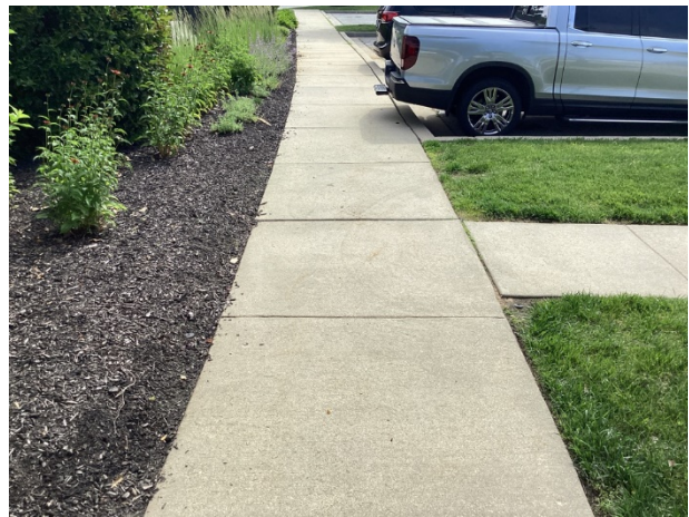
Concrete walkway sidewalk
