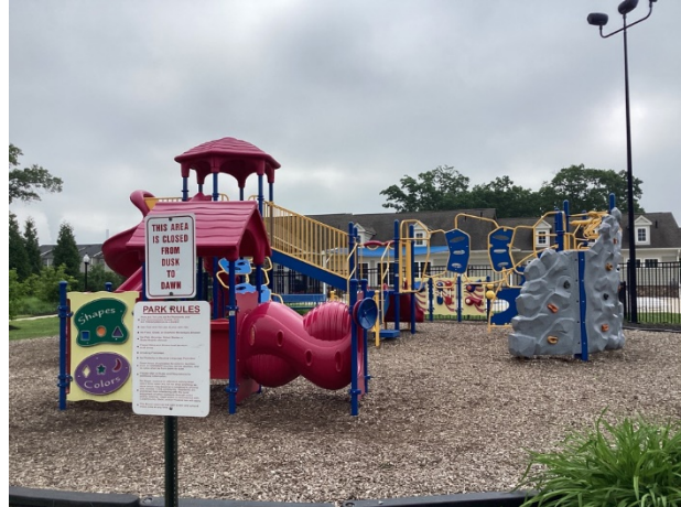
Clubhouse playground overview Note: Minor finish deterioration.
