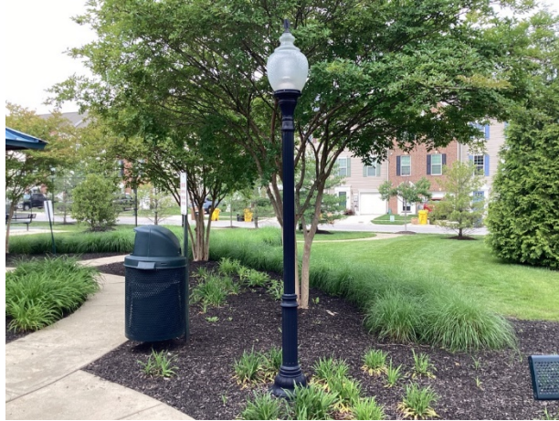
Light pole and fixture
