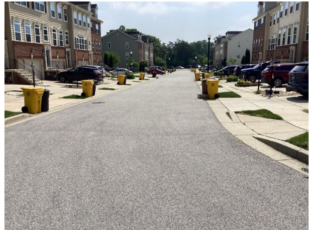
Section A pavement overview
