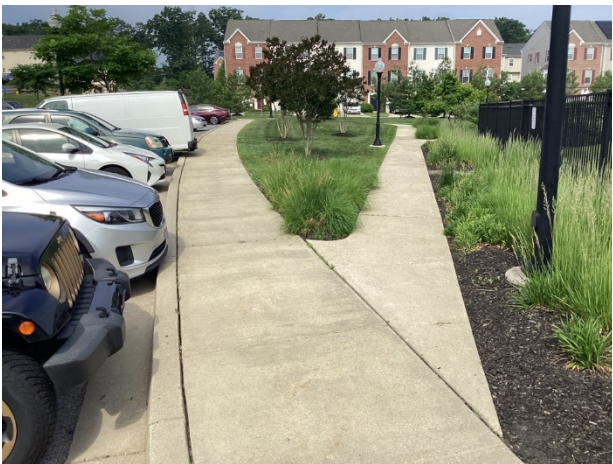
Clubhouse concrete sidewalks overview
